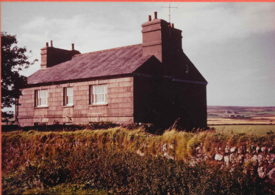
FARM HOUSE FROM ROAD. NOTE WALL AGAIN
