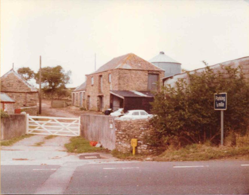
PORAT POLSTAIN YARD AND OUTBUILDINGS
